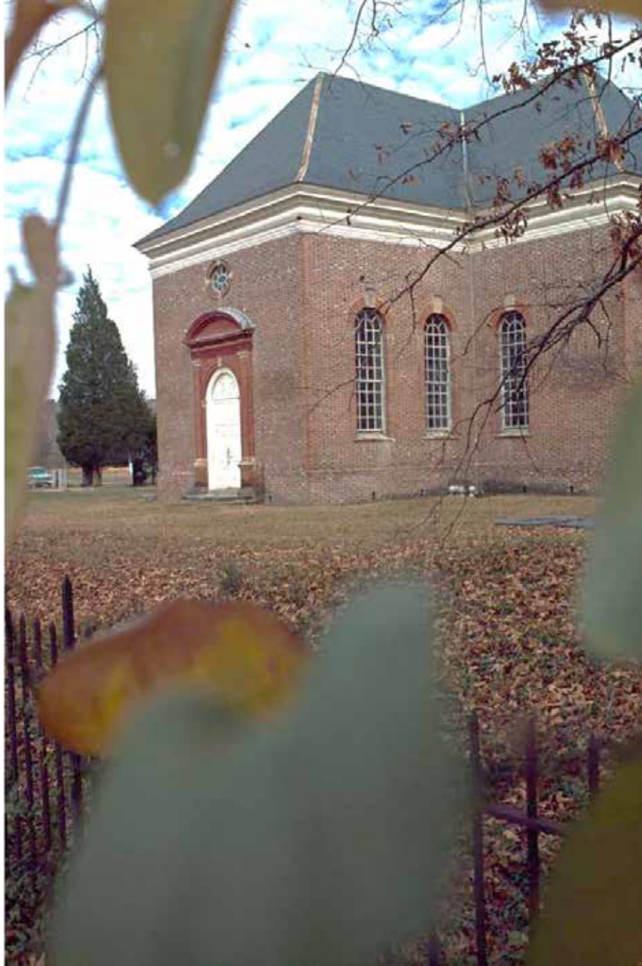
Christ Church Yard, southwest view c. 1960 Visible on the ground below the windows are the stone balls which once capped the brick wall that surrounded the Kelley plot. Note areas right (south) of west door and right of compass window that need repointing. Sheet metal rolls still on roof hips. Compass window to far left has stone sill wash running down brick wall. This is the only sill replaced on building (done in 1960s). One of the earliest color photographs of Christ Church and yard. From the FHCC Digital Images Collection .
