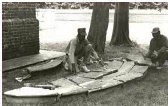
Stone Step repairs, 1974-1978
