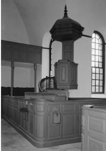
Christ Church Interior c. 1937 The Historic American Buildings Survey (HABS) captured Christ Church's pulpit in this photograph from 1937. Note the donation box mounted under the clerk's desk at the crossing (right) and the guest register stand mounted on the other side (left). Visible along bottom of pews is copper flashing installed as termite and water protection in 1933 during repairs to pews/floor joists carried out by Claiborne & Taylor of Richmond.
