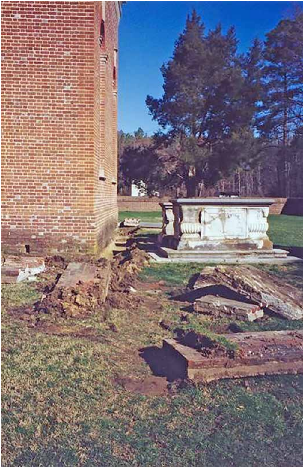
Splash Removal 1997 The brick splash installed c.1967 proved ineffective at mitigating rising damp (besides being historically inaccurate.) Note the cant of the placement of the tombs.
