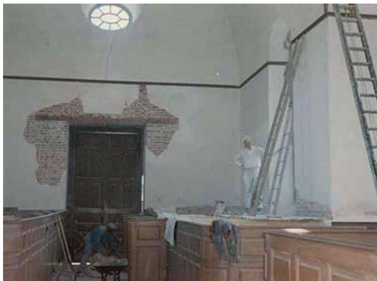
1965 north door and northeast wall plaster repairs
